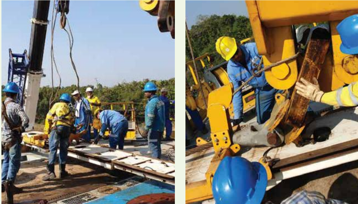
Rig Building Activities
