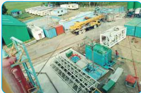
Typical Drilling Field Constructed by Construction Division
