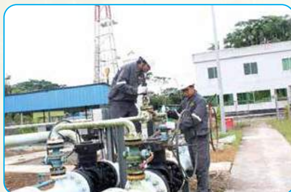
Gas Process Plant Maintenance by BAPEX Engineers
