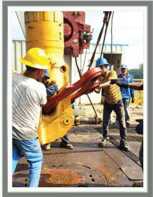
Drilling activity on the Rig Floor
